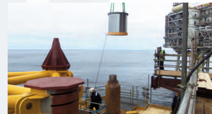
◀ Preparing to install one sleeve onto the column
